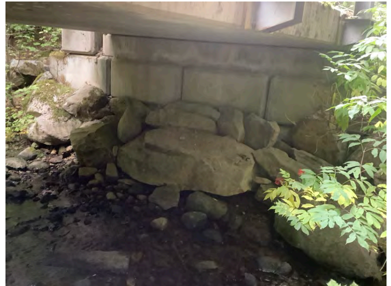
Left Bank Abutment when facing downstream
