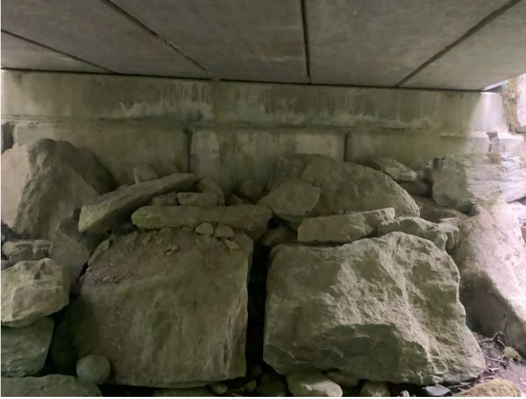
Right Bank Abutment when facing downstream
